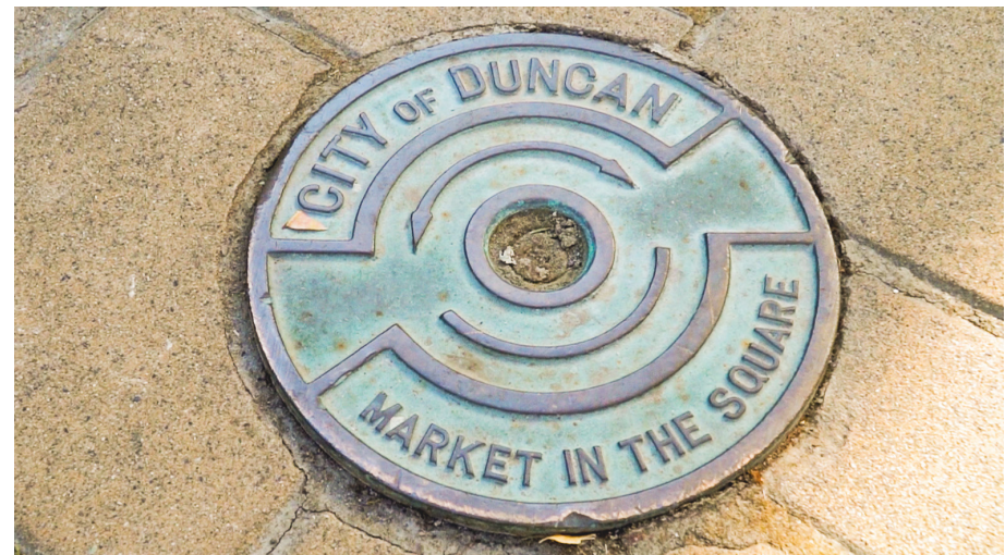
Bollard cover on the perimeter of a town square that can be closed to cars for community events.
