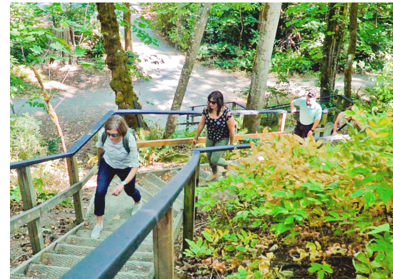
This staircase provides a direct connection for pedestrians across a steep grade between the trail below and the road above.
